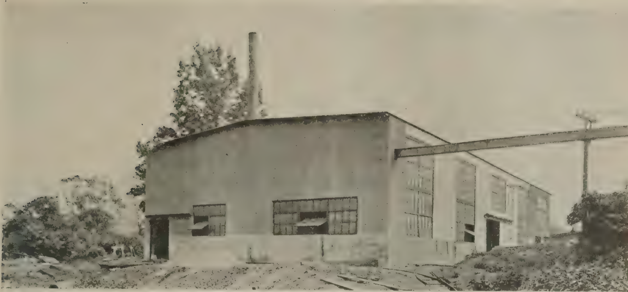
New building, Porete Manufacturing Co., Newark, N. J. E. Walter, Designing Engineer
